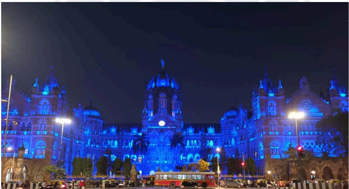
Night view of CSMT station celebrating 100 Years of Electrification
