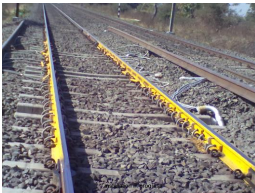
Instrumented rails on up main line
