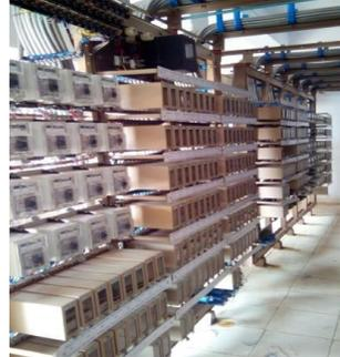
2. Replacement of SM's slide and overhauled indoor signaling gears along with provision of push button control panel commissioned at Tinkheda station on 15.06.2017.
